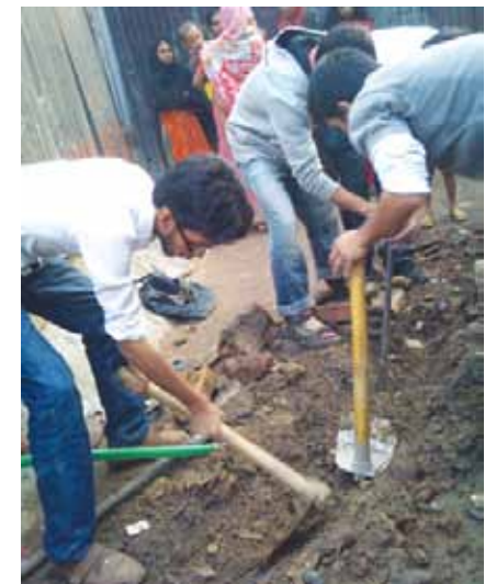
BBLT 5 participants repair a faulty water system in Korail.
